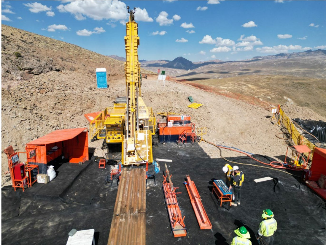
FIGURE 2: DRILL RIG ON SITE AT COBREMANI TARGET.
